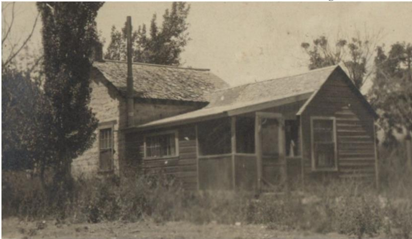
The old Annie Clark home where Myral was born and raised. The concrete room is on the left. The wooden additions are on the right. Photo taken in 1917
