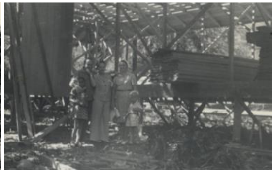
The new house begins to take shape
