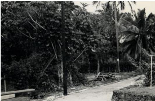
Construction of the new house began Aug 12, 1941
